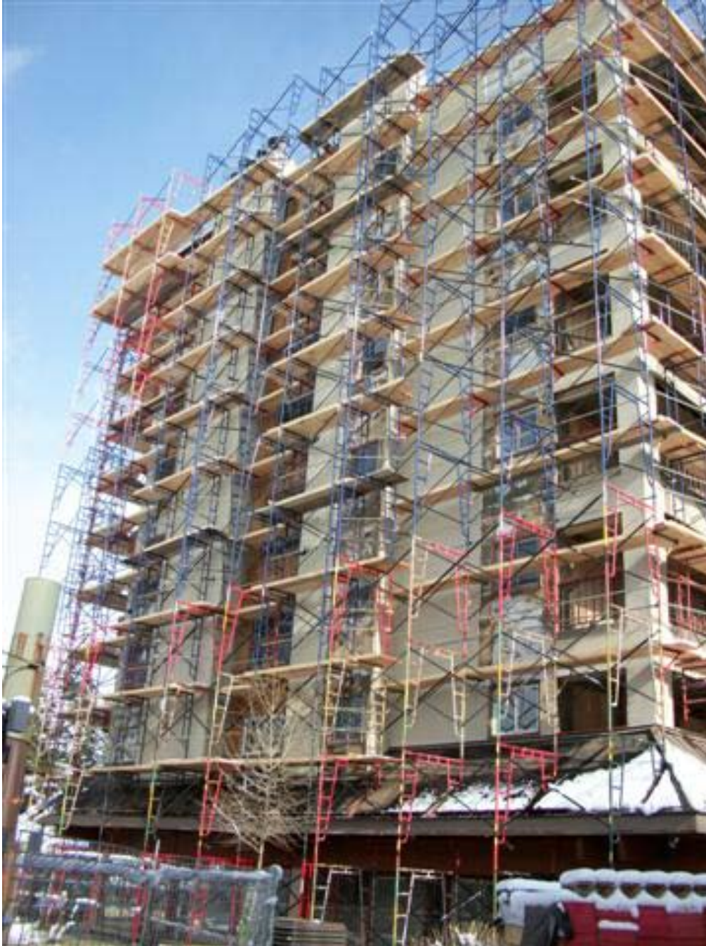
View of East side of Plaza 2 w/ Scaffold complete
