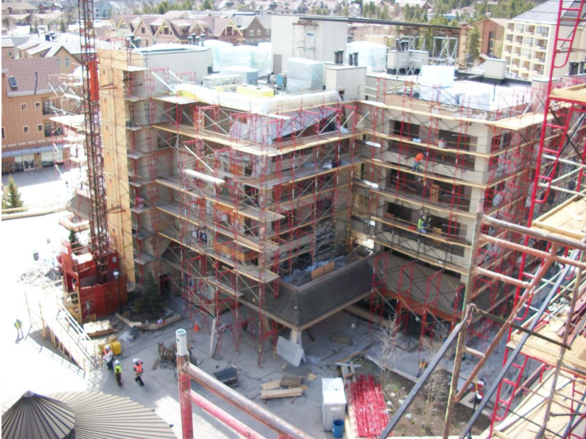
View of North & West sides of Plaza 1 taken from atop Plaza 2
