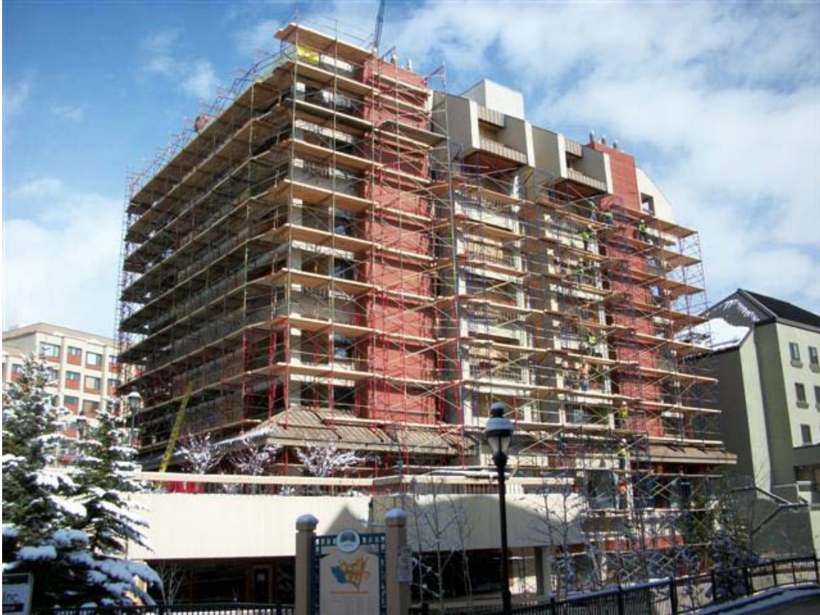
View of East Side of Plaza 3 showing scaffolding nearly complete
